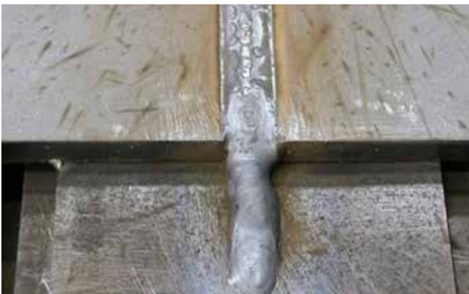
Figure 24 Pay attention to the stops, which are placed on the sacrificial plate. This plate is then removed by grinding.
